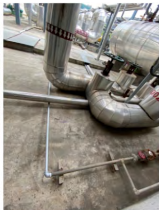
Reconstruction of Steam Condensate Collection in Plant Area
