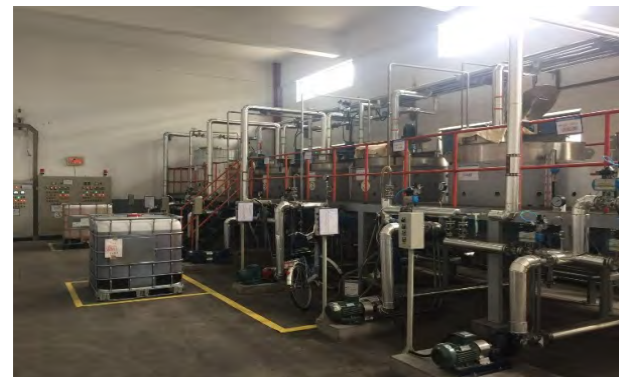
Raw materials are delivered in a closed pipeline system to prevent the fugitive diffusion of volatile organic waste gas and dust.
